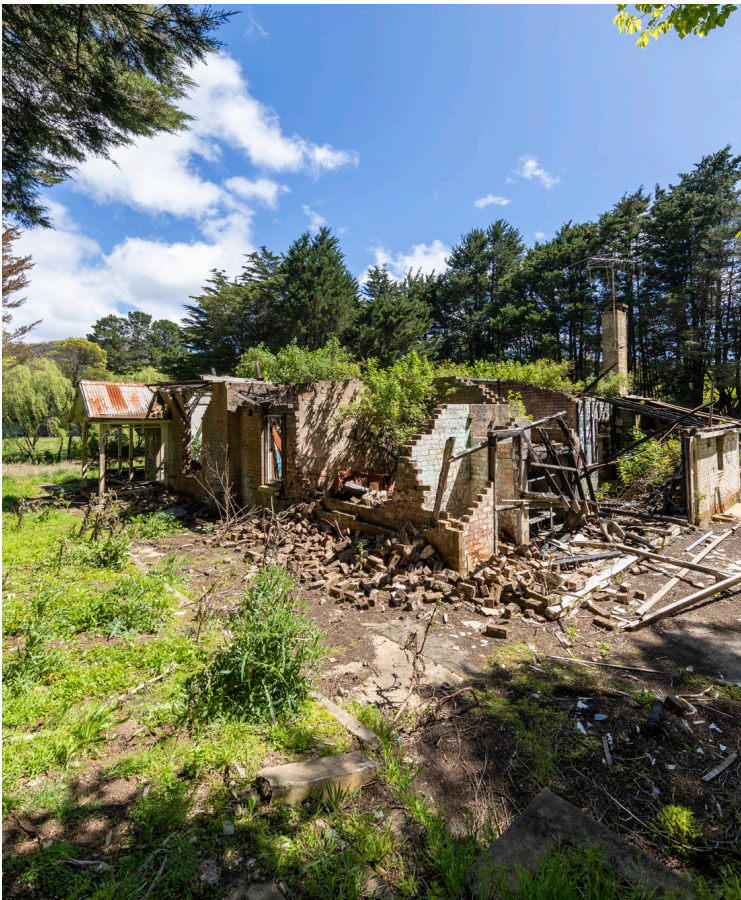
Existing site photos illustrating the current conditions.
