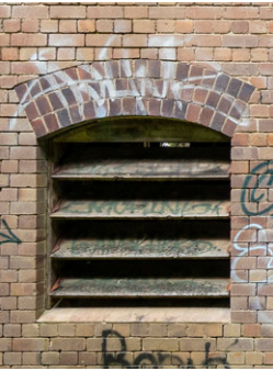
Timber Louvers re-stored and new
