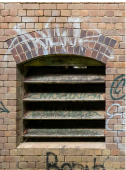
Timber Louvers restored and new
